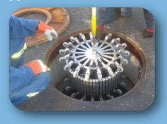
The tools can be directly loaded into the pipeline through a manhole or an open pit, or they can be inserted through a manhole in smaller modules and assembled inside the manhole chamber. The Chimera tools can either be tethered on both ends and winched through pipeline sections up to 6,000 feet or where conditions allow, they can be deployed in a free-swimming mode and travel longer distances between access points.
