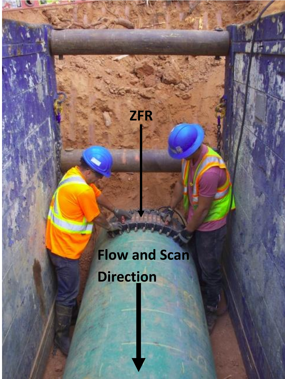
Figure A2-2: Typical initial location of the Bracelet™ Probe placed at the start location.
