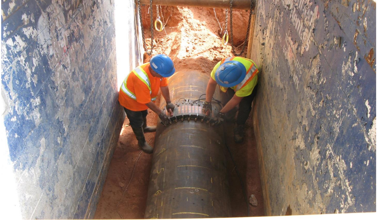
Figure A2-3 Typical BP scanning a pipe.
