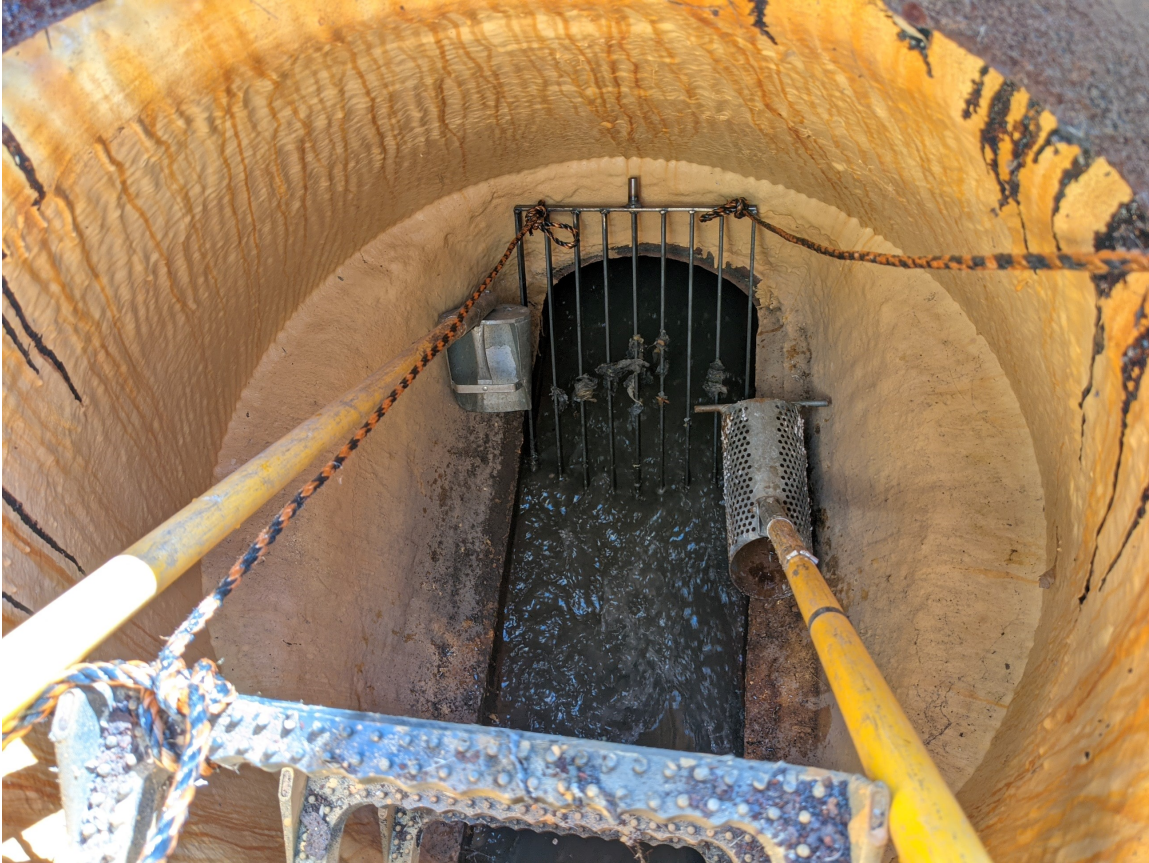
Fig-7: screen to stop Navigator and scoop to retrieve it.
