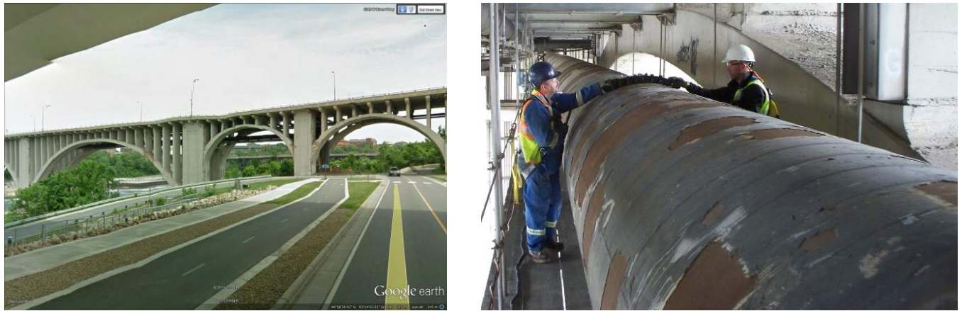
Figure 4. Street view of 10 th Avenue Bridge (left) and scanning of 54” pipe under bridge (right)
