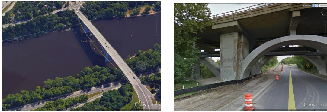
Figure 1. Franklin Avenue Bridge, from above and street view (Google Earth)
