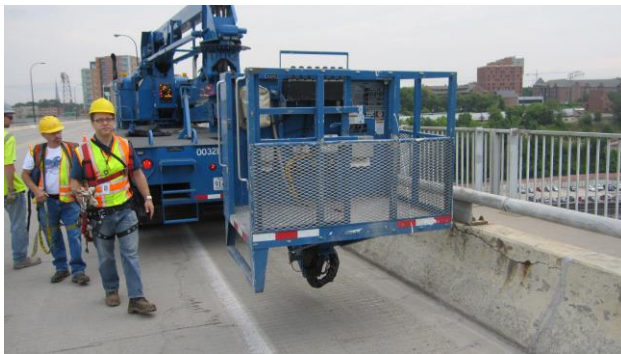
Fig 7. Snooper truck used for access to the planked walkway.
