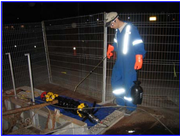
• Figure 2. Tool Sanitization before job
