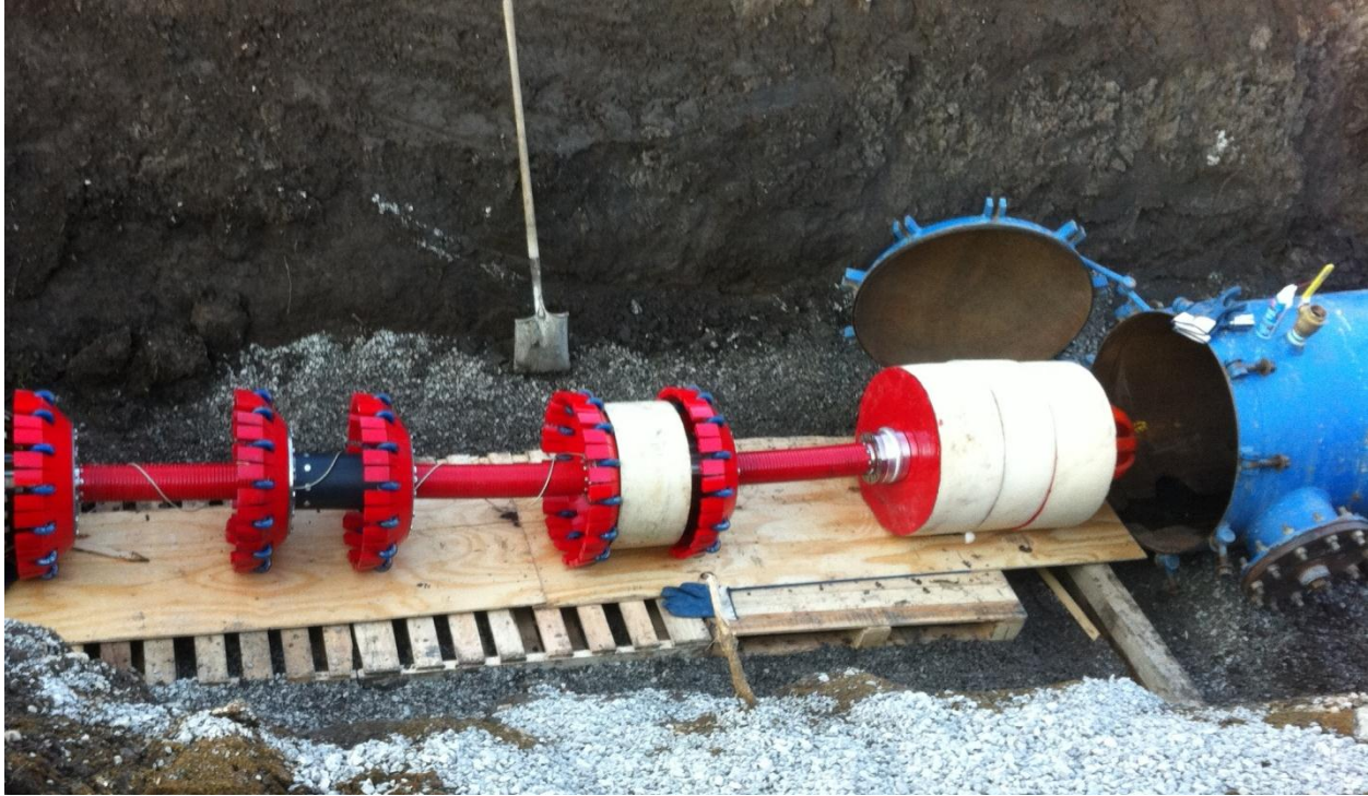
Figure 2. Picture of 24" SeeSnake tool (Pre-inspection)
