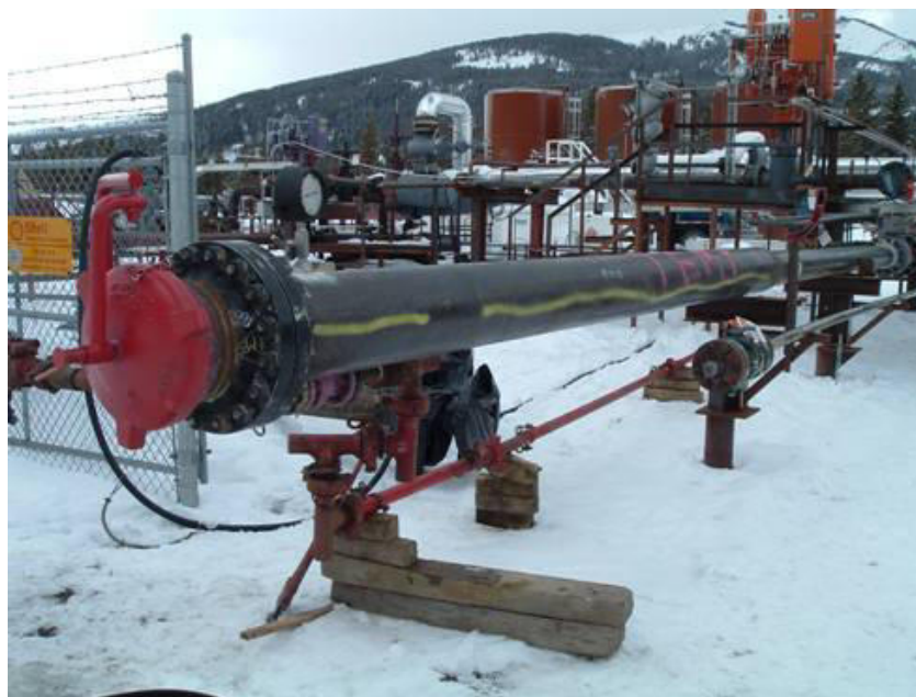
Fig-4: Typical launch barrel for O&G application
