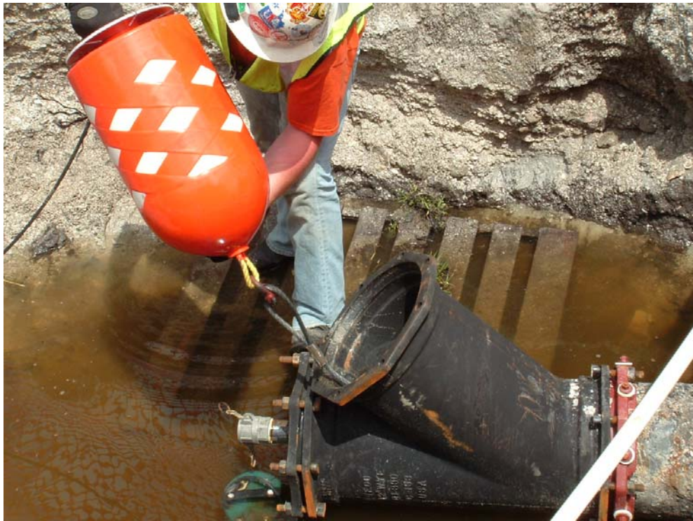
Fig-4: Pre-cleaning the line (cleaning and sizing pig is winched through)
