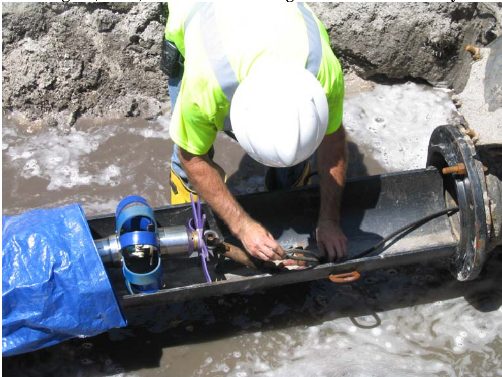
Fig-2: Wire rope being attached to Tool
