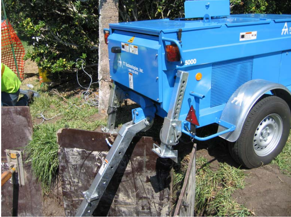
Fig-3: Winch unit being used to pull tool
