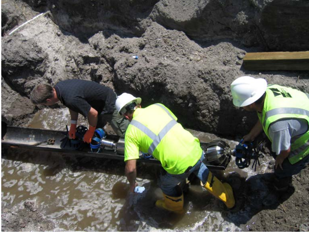
Fig-1: (above) 12” PICA Tool being loaded into launch tray
