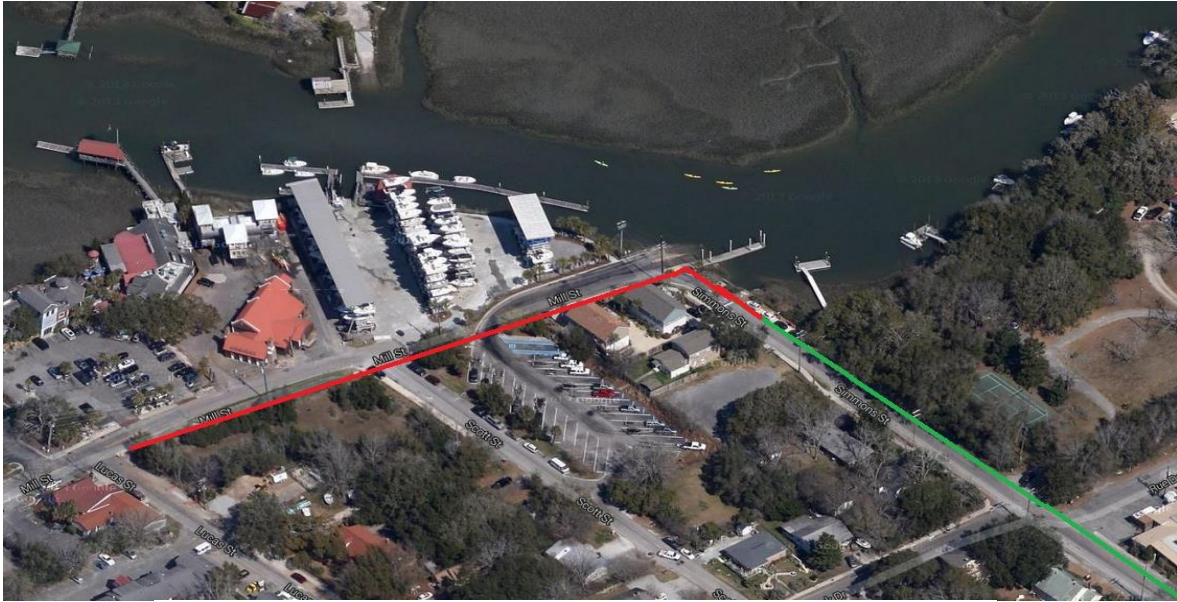
Figure 6: Google Earth view of the 16" Simmons Road Force Main. The red section identifies pipe that is highly corroded; the green section identifies pipe that experienced minimal corrosion.
