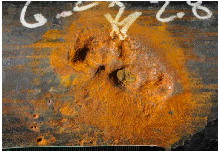
Figure 11: Through-Wall External Corrosion Pit from CML Pipeline.
