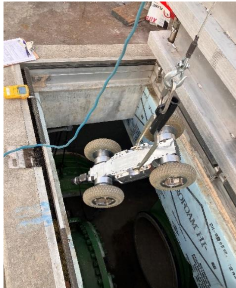
Figure 4 - VC7501 PICA lowering down robotic crawler equipment.
