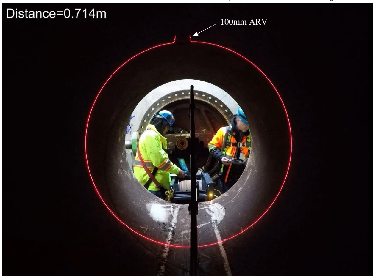
Figure 28 - Laser projection ring on the pipe wall at 0.714 m from Zero Reference Datum (ZRD) VC7501
