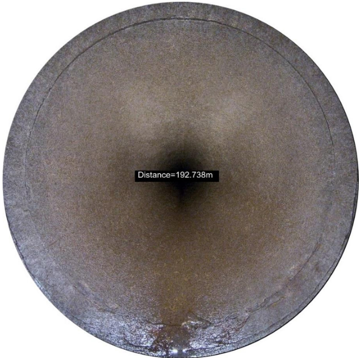
Figure 17 – Sample observation of minor grout cracking at joint
