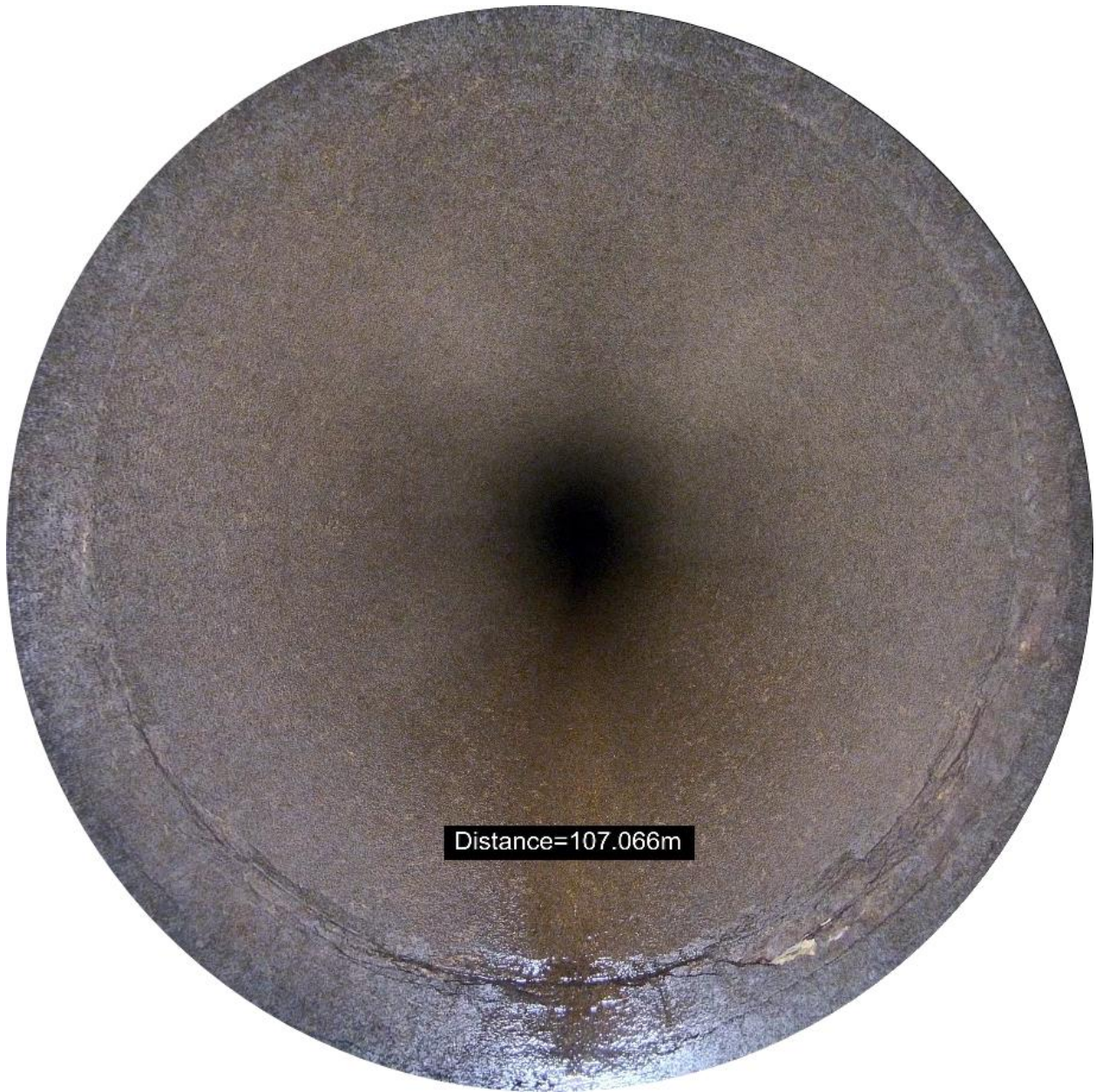
Figure 18 – General observation of the grout cracking at the pipe joint with minor spalling
