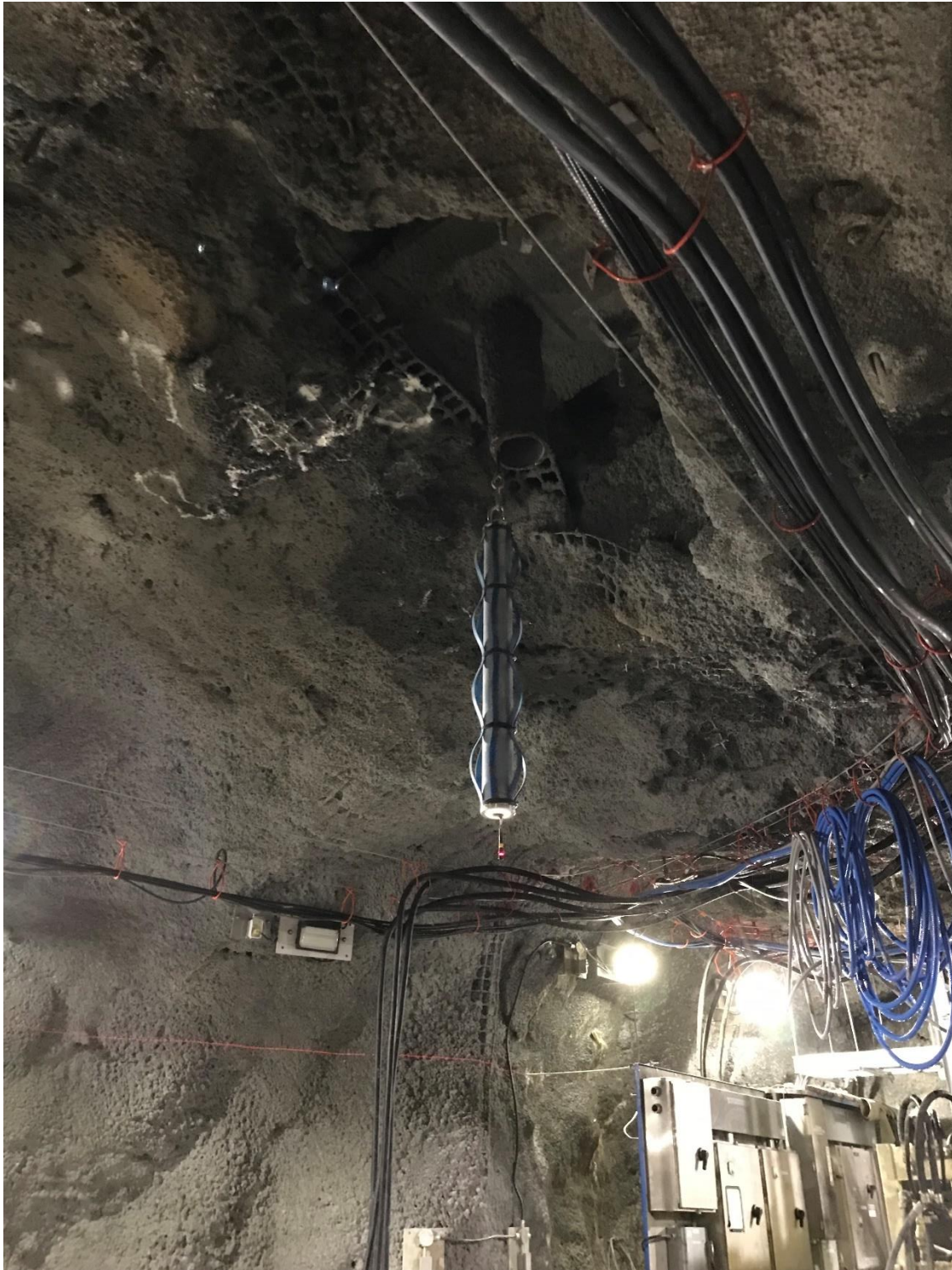
Figure 10. Laser tool exiting at 530 meters below inside mine corridor
