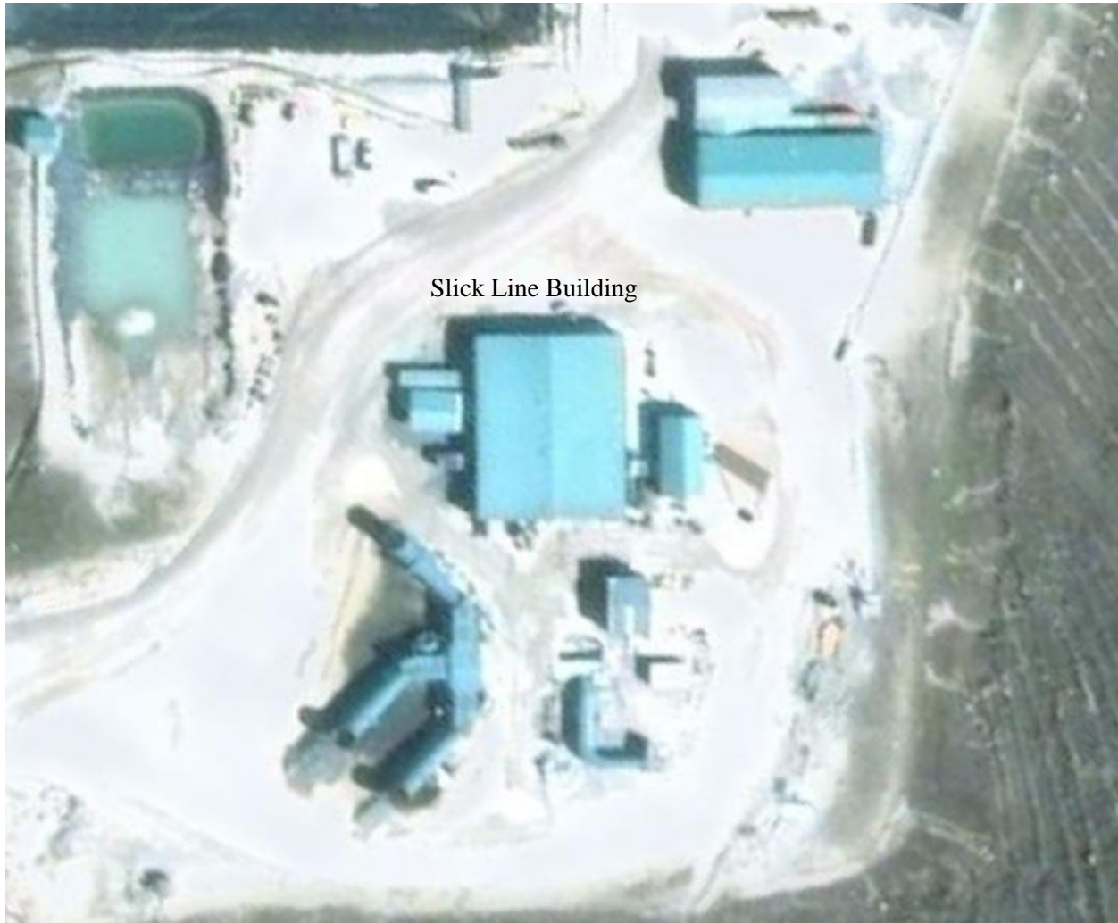
Figure 4. Google Earth Map – Slick Line Building Location
