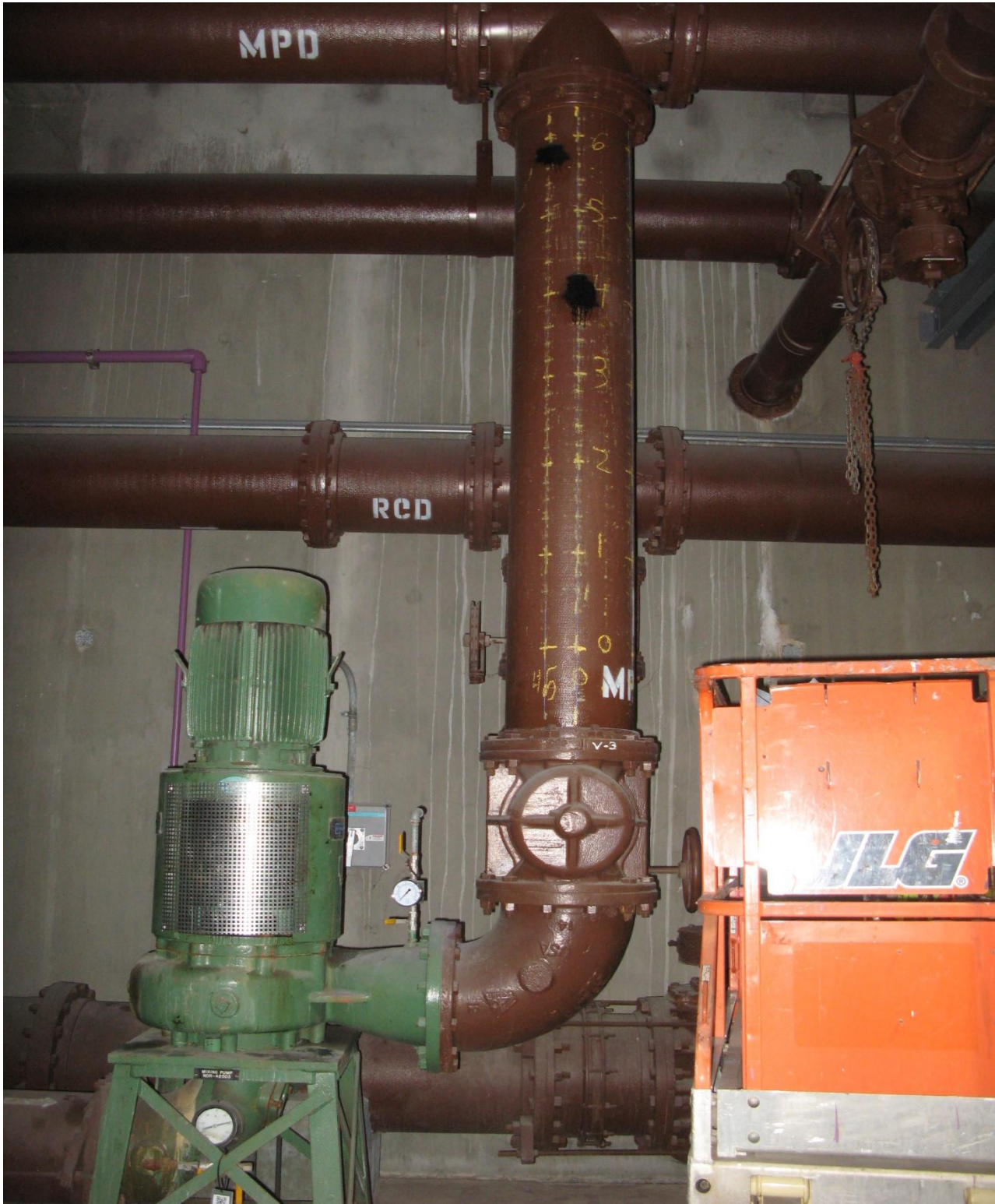
The picture above shows an example of the Vertical Discharge piping.
