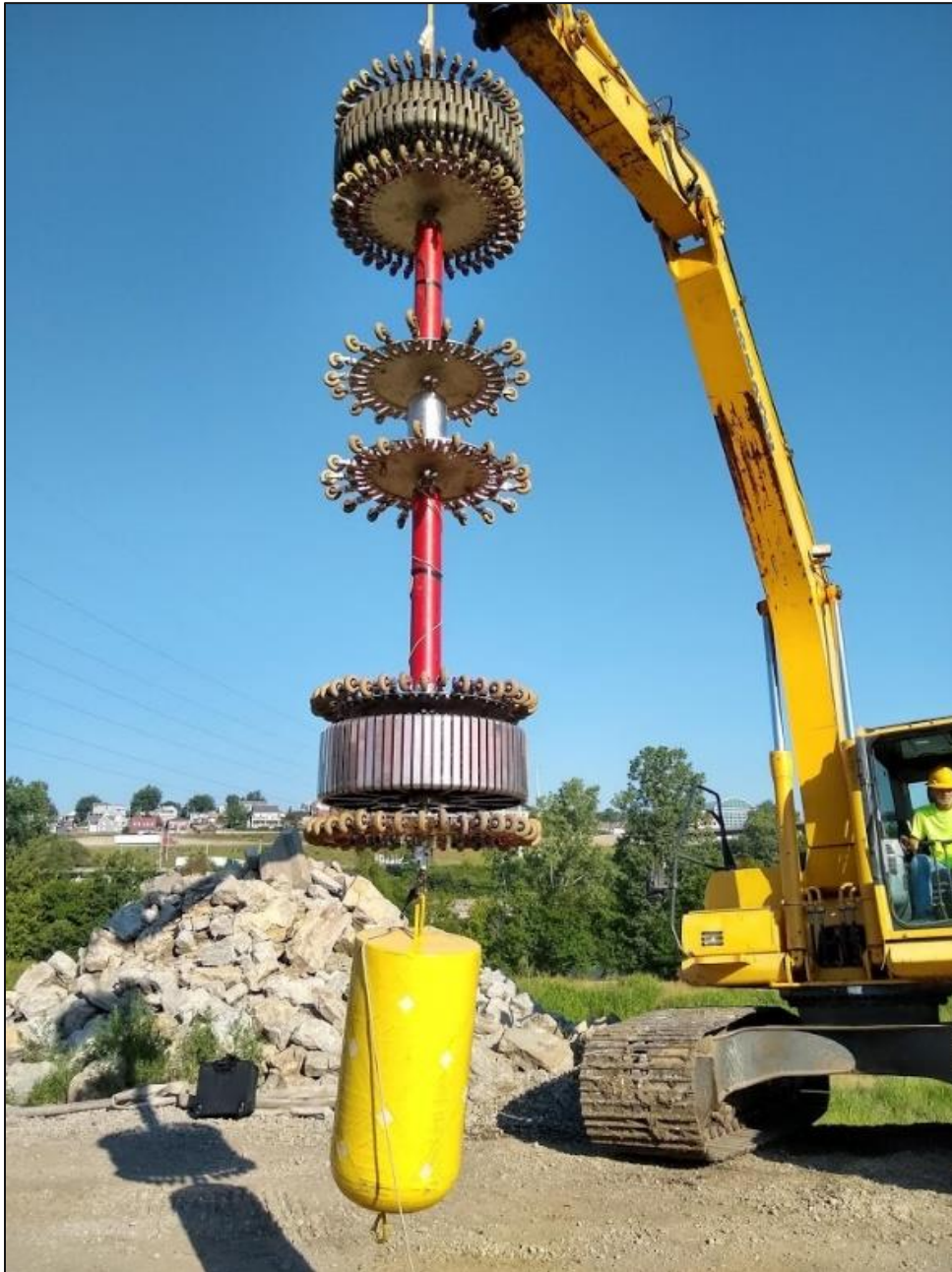
Figure 3: PICA’s 36” Chimera prior to inspection of the South force main.
