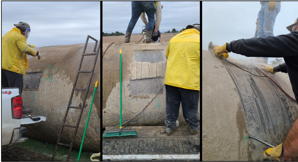
Figure 3. PICA technicians removing an outer concrete window
